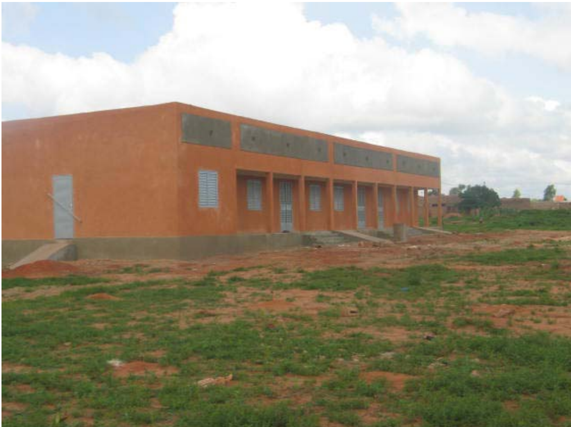
One of the new school buildings with 6 classrooms.
